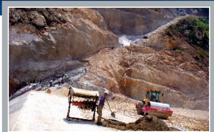
Simultaneous operation of left plinth formwork, preparation of dowel execution, compaction of body rockfill layer and instrumentation cable protection
