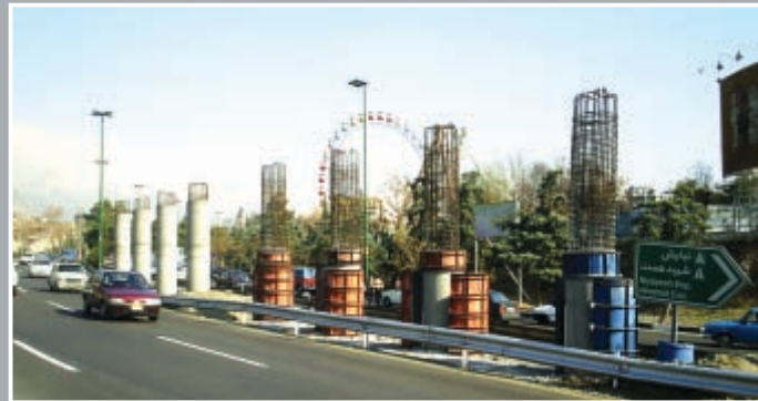
Construction of bridge pier and head in heavy traffic
