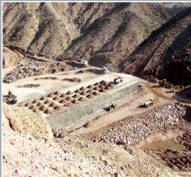
Construction of cofferdam - soil cement type
