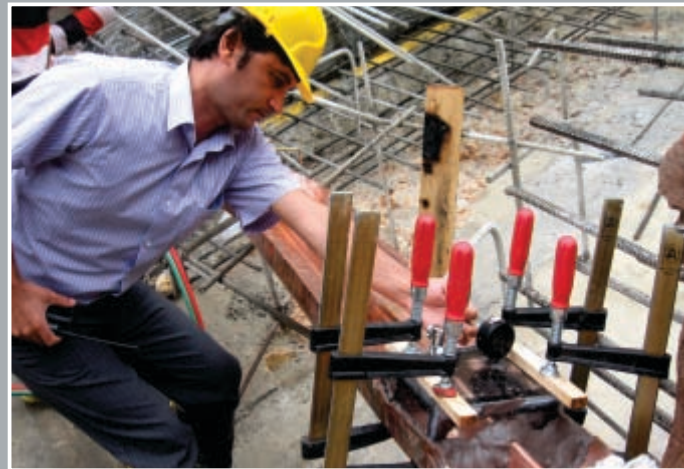
Copper water-stop execution
