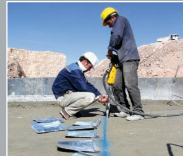
Construction of contraction joint
