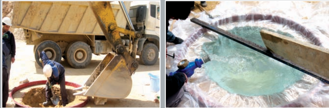
Compaction and permeability test
