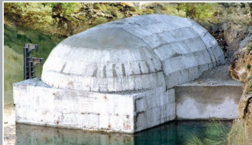
Submerged intake structure
