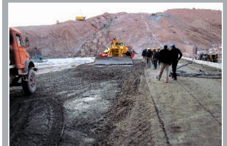
Construction of roller compacted concrete
