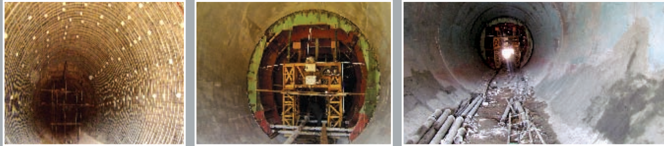
Construction of diversion tunnel lining
