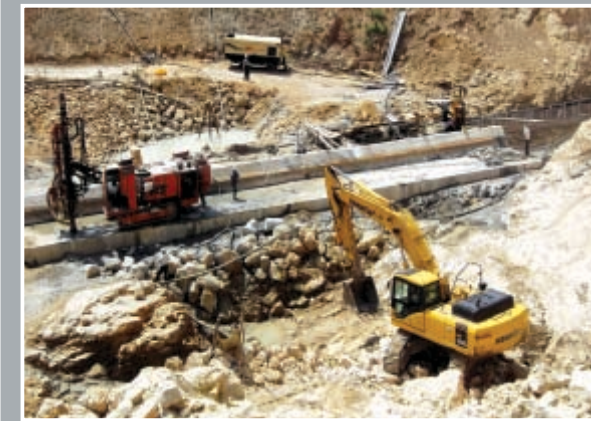
Middle plinth reinforcement
