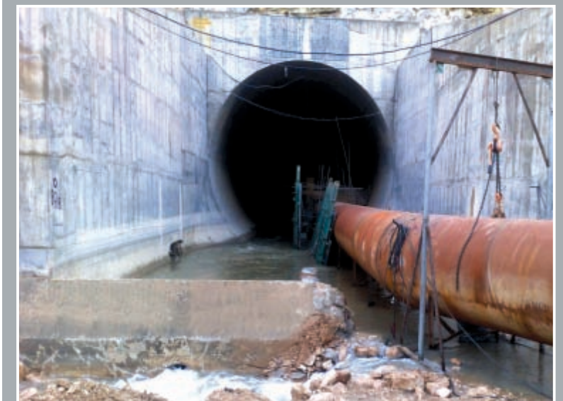
Installation of intake pipe within diversion tunnel
