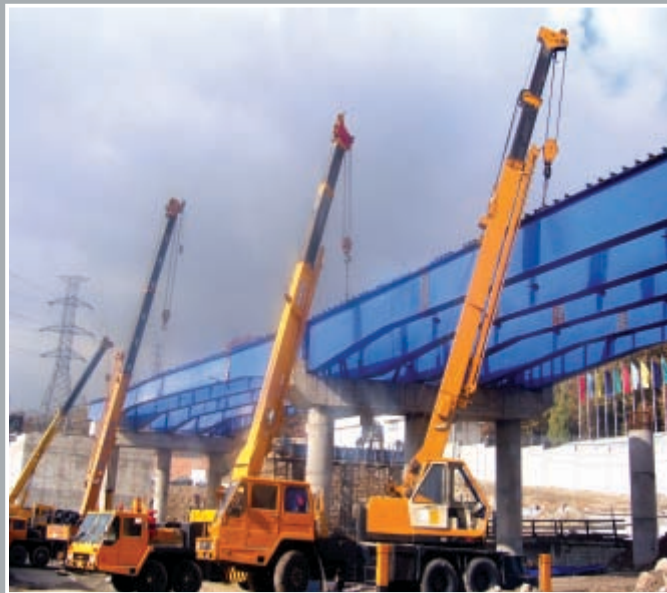
Installation of metal decks of the bridge in two shifts due to heavy traffic
