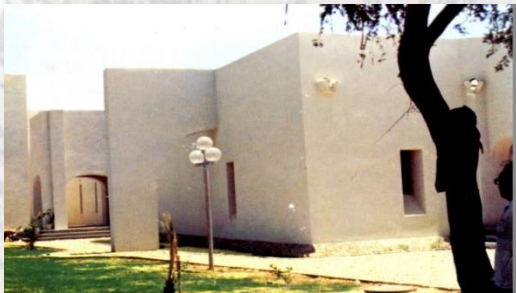
Bandar Abbas TV broadcasting centre
