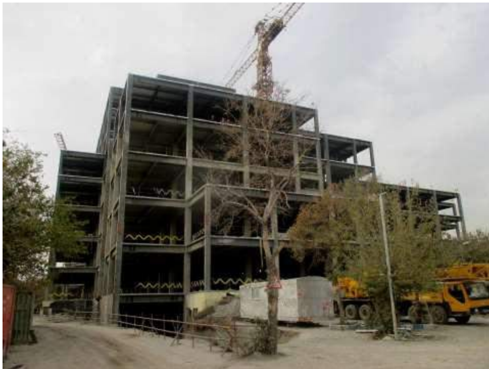
Structure Of Farabi Hospital
