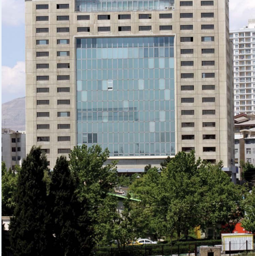
Ministry of Science, Research and Technology Building
