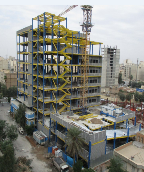
The Management Building Of Tejarat Bank Branches - Khuzestan Province
