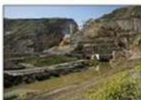
Seymareh Dam Diversion Tunnel
