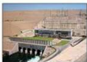
Karkheh Storage Dam HydroPower Plant
