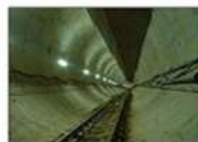
Tehran Metro Underground Railway (Mehro)
