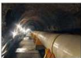
Semnan Water Supply Tunnel
