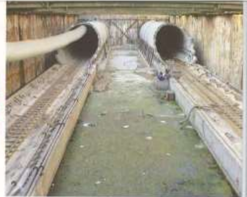
Concrete TBM cradles
