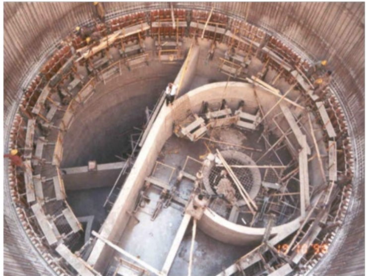
Tehran Khayam Tunnel Project
