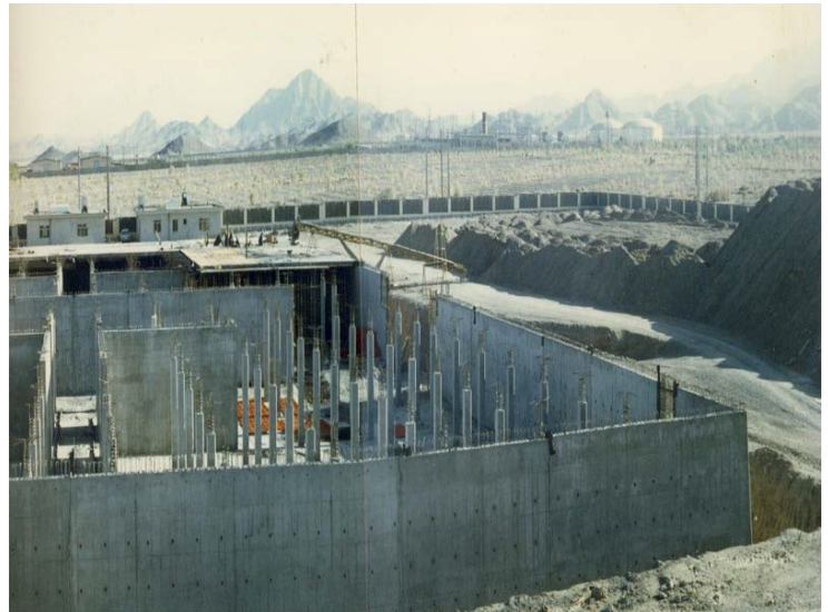
Zahedan 30.000-Cubic Meter Reservoirs
